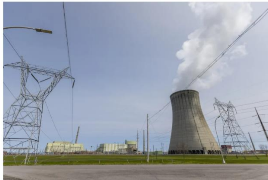
A cooling tower at a nuclear station in Scriba, New York. Photographer: Lauren Petracca/Bloomberg
