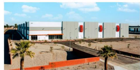
Meyer Burger's existing module plant in Arizona will now be supplied by the company's German cell facility.
