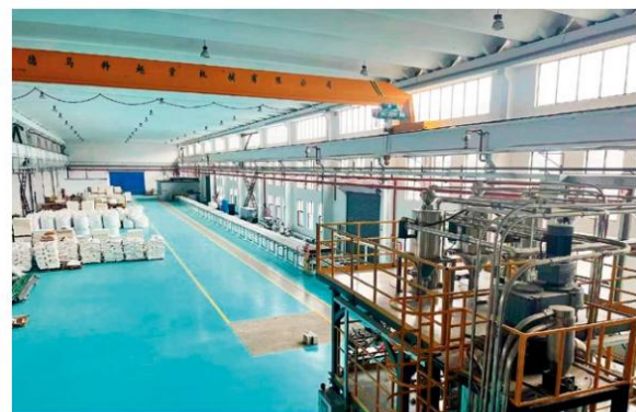
CR Chemical Materials' PET foam production line
